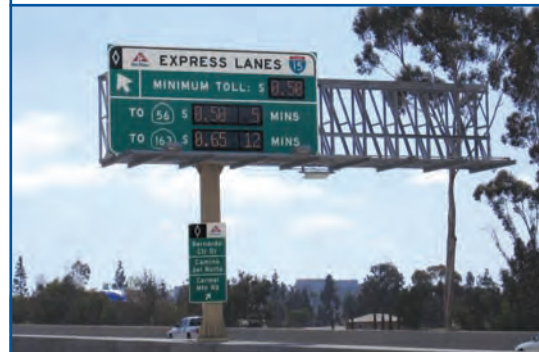
HOT Lane Installation San Diego, California
