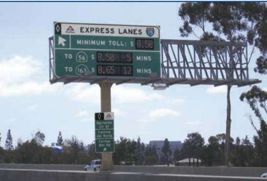
HOT Lane Installation San Diego, California
